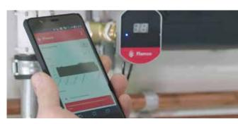
The optional Flexcon PA App is handy when initially filling the central heating system. The app provides insight into the central heating system's pressure history.
