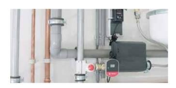
The Flexcon PA AutoFill monitors the pressure in the central heating system. With a permanent connection to the water pipe, the system is automatically topped up to the required pressure level whenever it drops.
